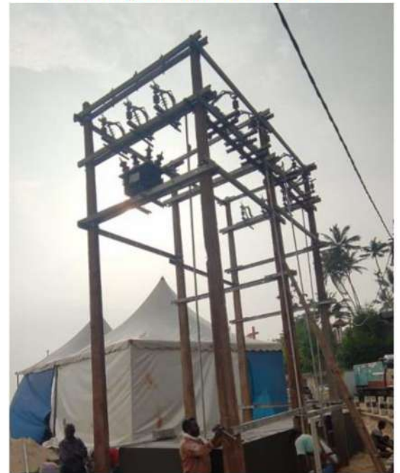
Standard plinth set up for installing multiple transfofmers.
